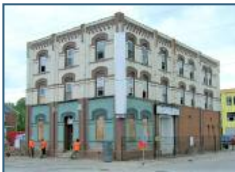
Then: Restoration begins in the summer of 2009. The painstaking removal of paint from the brick exterior of the old hotel was a turning point for the new owners. For more on cleaning historic masonry, see Page 4. Photo courtesy of Rick and Anke Lex.
